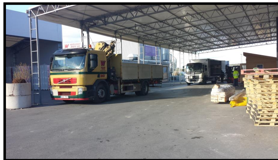
Loading bay – Construction Consolidation Centre
